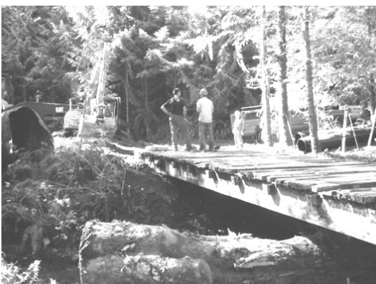
Railcar bridge installed to replace the undersized culvert at Shirley Creek.
