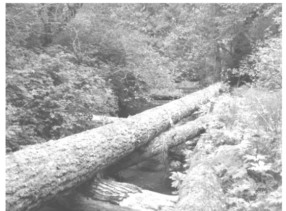
One of the complex large wood structures designed by Habitat Consulting LLC., placed as part of the Condon Creek Restoration Project.
