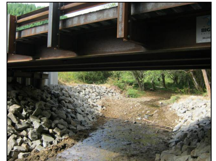
Swamp Creek After Bridge on Swamp Creek after culvert removal in 2011
