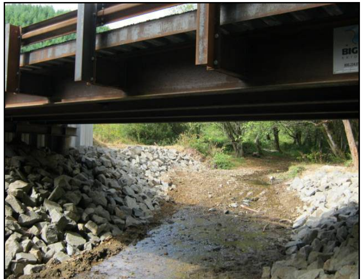
Swamp Creek After Bridge on Swamp Creek after culvert removal in 2011
