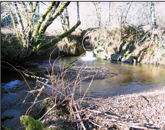
Swamp Creek Before Culvert on Swamp Creek before removal in 2011
