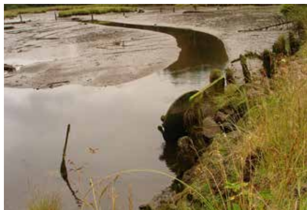
Tidegates like this one play an important role in supporting agriculture in the tidally connected areas of the lower river. Many tidegates are being replaced to improve fish passage and water quality behind the gate.
