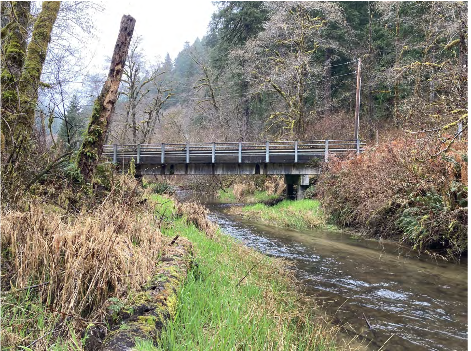
Downstream of bridge looking upstream (2/27/2024)
