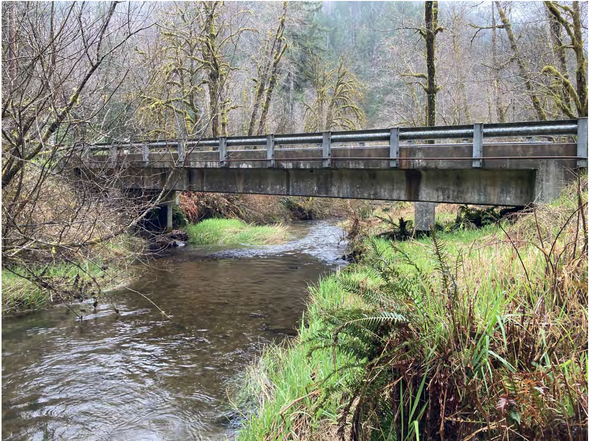
Upstream of bridge looking downstream (2/27/2024)
